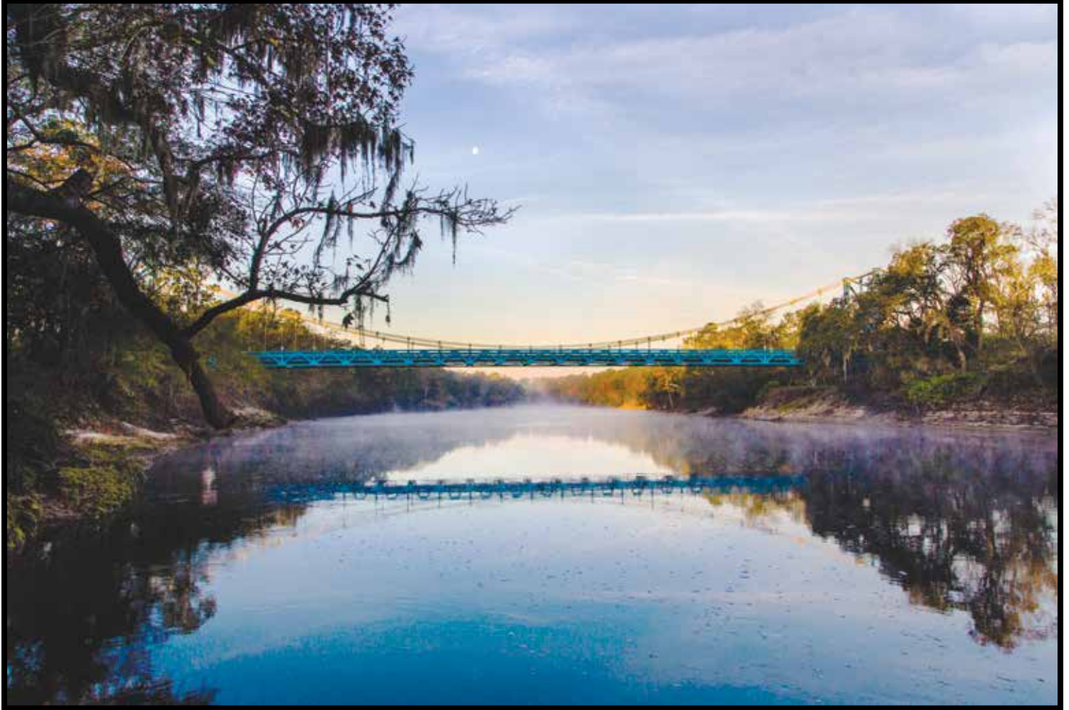
Hal Adams Bridge Over the Suwannee River, Lafayette County: the oldest suspension bridge in Florida. Credit: Mr. Jack Howdeshell
